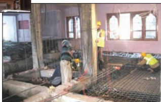
Retrofitting work in progress Inset: Building to be retrofitted
