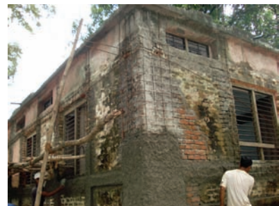
Retrofitting in progress
